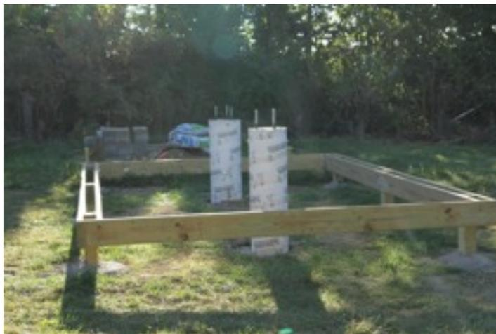
On Friday August 27th, we poured the footings for the buildings and the piers for the telescopes. I have been looking forward to getting the concrete poured for two reasons. First, it means that the YRS site is ready for the move. Second, we are past the heaviest labor of the project.
